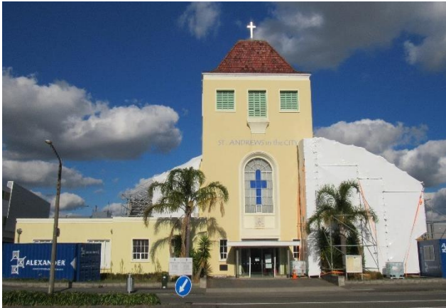
Renovating St Andrews
